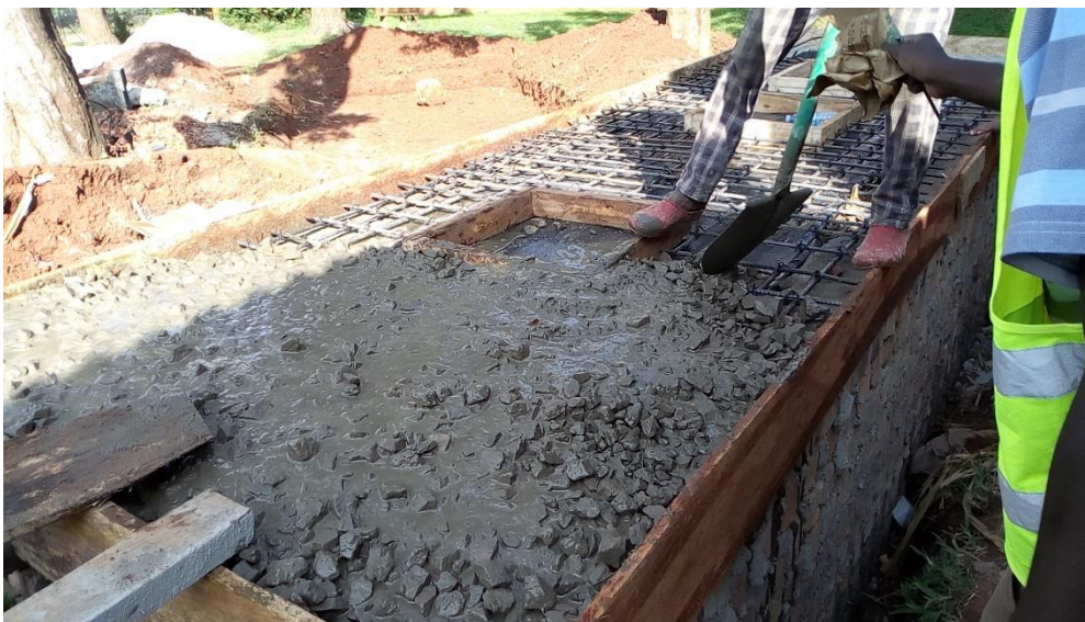
Figure 16: Casting of ABR top slab
