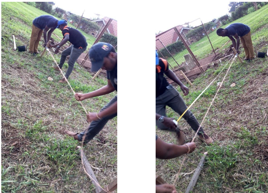
Figure 10: Setting out activities
