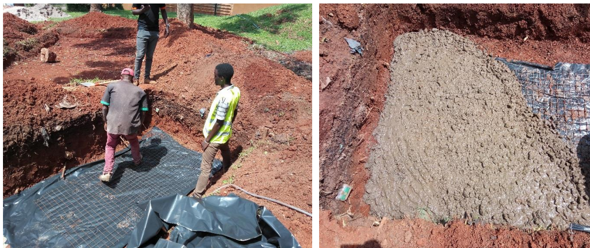
Figure 12: Casting of blinding concrete
