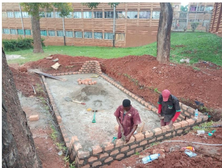
Figure 13: Brick wall construction
