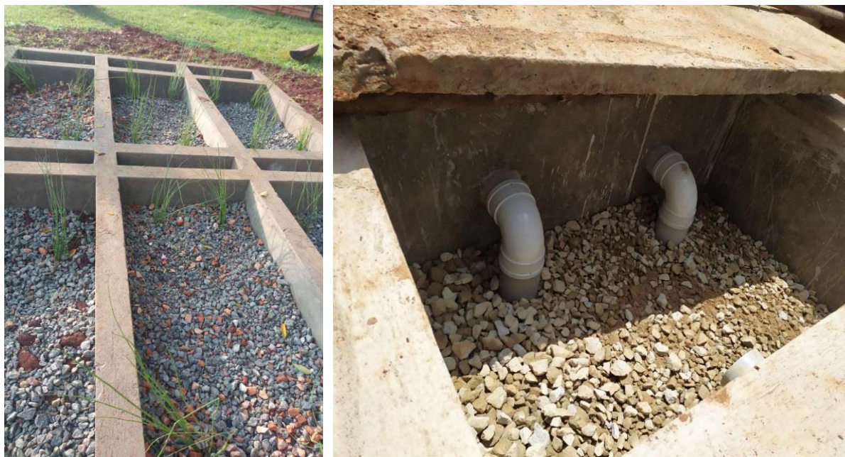
Figure 17: Substrate in Anaerobic filter and constructed wetland
