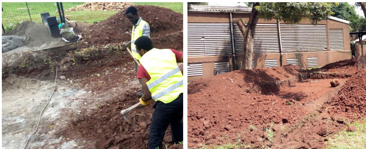
Figure 11: Excavation of site
